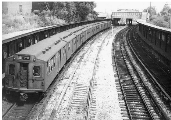
Photo 1.23 New York City rapid transit train of the Brooklyn-Manhattan Transit Corporation, built ca. 1936 (Courtesy of William D. Volkmer collection)
