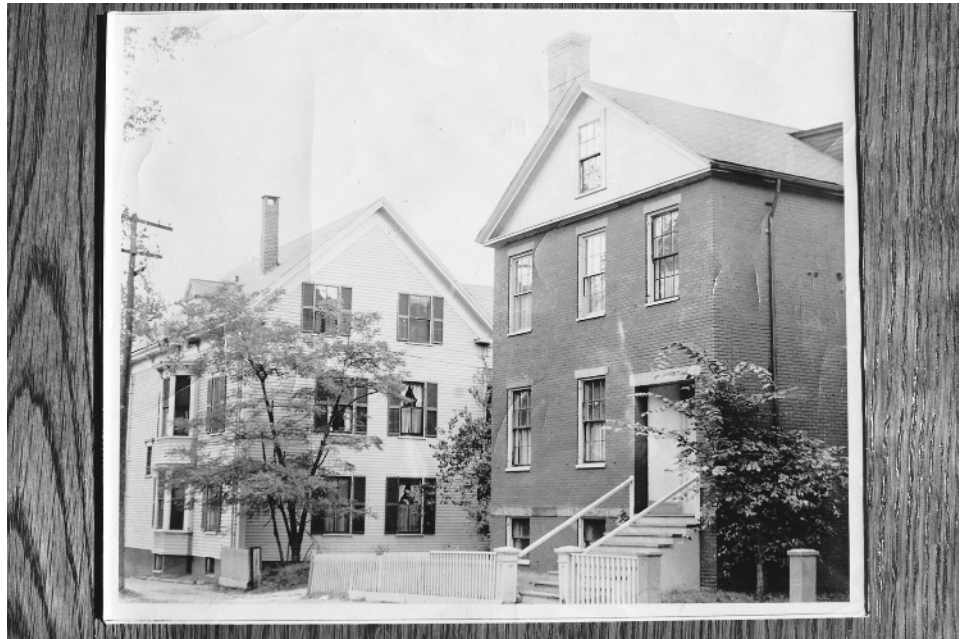
Figure 1-4 Research can reveal historic photographs of a building that can be used to confirm materials or details that have changed through time. This photograph shows the appearance of a Federal period house prior to addition of a later porch that changed the original entrance.
