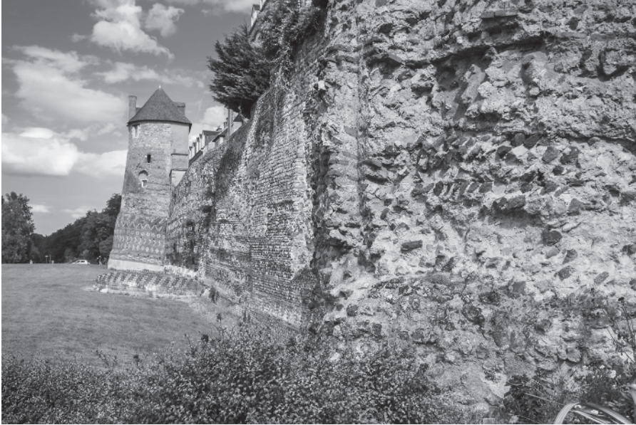
Figure 1.2 Roman wall, Le Mans. As the northern empire became unstable, city fortifications were strengthened, and extraordinarily durable walls like this one survive quite widely, as in Colchester.
