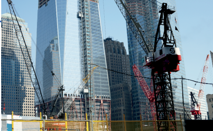
Construction on One World Trade Center.
