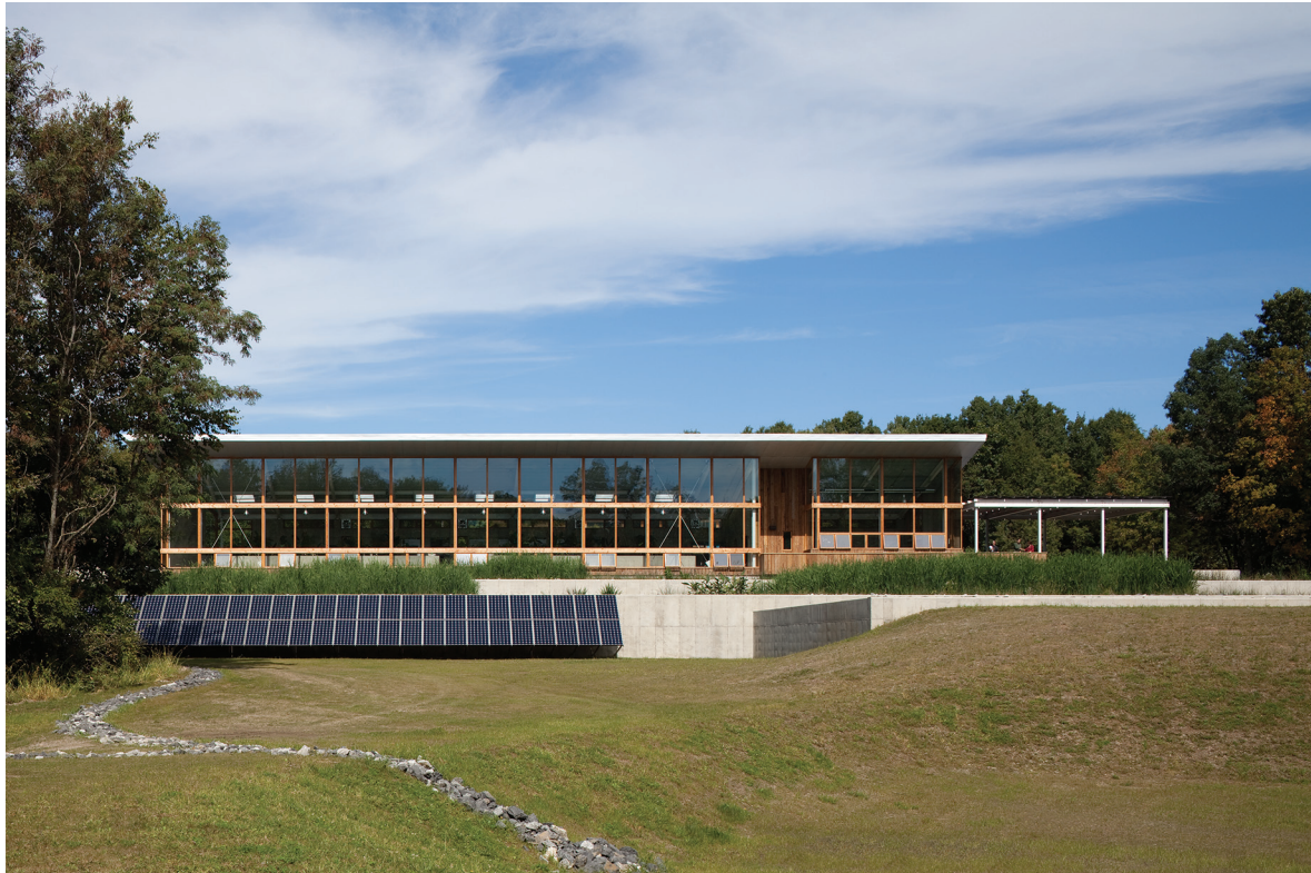
■ FIGURE 1.3 The Omega Center for Sustainable Living is net zero energy and one of the world's first certified Living Buildings. Image courtesy of BNIM; photograph © 2009, Assassi.
