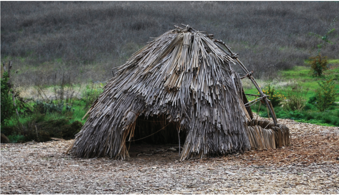
FIGURE 1.5 Basic shelters use natural forms of grasses and thatch as design elements to protect the occupants from rain and wind.
