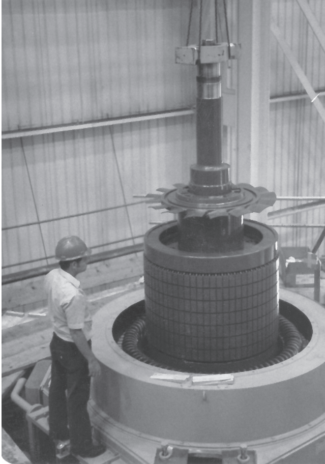
Figure 1.1 Photograph of an SCI rotor being lowered into the squirrel cage induction motor stator.
