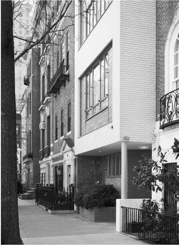
Figure 1.21: Edward A. Norman House, 124 East 70th Street, New York, New York. William Lescaze, 1941. The thin column, the wide, horizontal openings, and the shallow brick veneer of the Lescaze house all emphasize that the facade is a curtain wall rather than a structural, load-bearing wall. That is one of the reasons why the house has a different effect on the streetscape than the neighboring houses.
