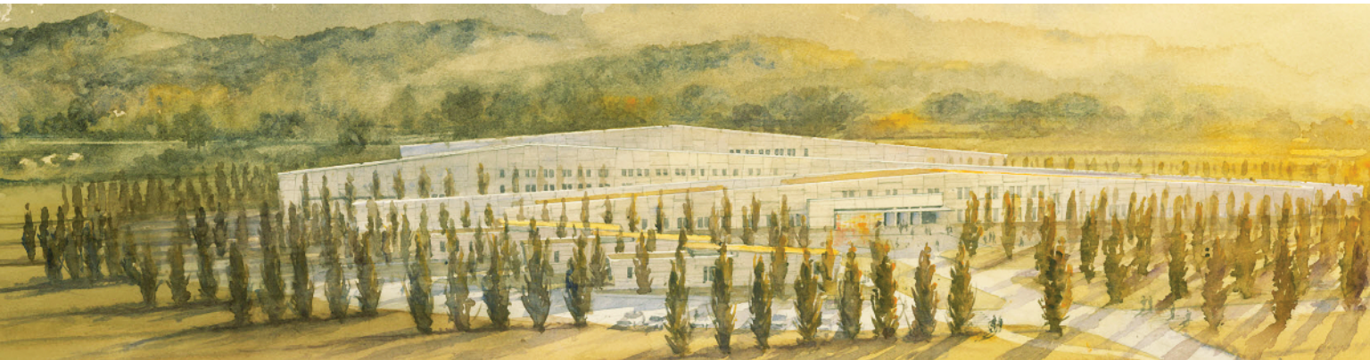
Figure 1.6 Oregon State Hospital at Junction City is designed to meet the 2030 Challenge 2015 goal. Source: HOK
