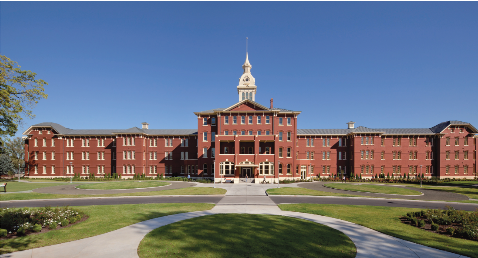
Figure 1.5 Oregon State Hospital at Salem, Oregon, is designed to meet the 2030 Challenge 2010 goal. Source: HOK with SRG Architects
