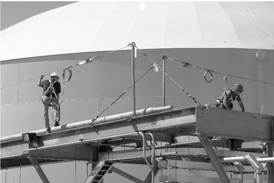
Figure 1.9 Multiple, complementary horizontal lifeline systems. Credit: Reliance Industries, LLC.
