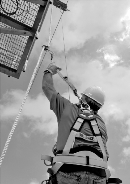
Figure 1.7 Vertical lifeline system. Credit: Reliance Industries, LLC.
