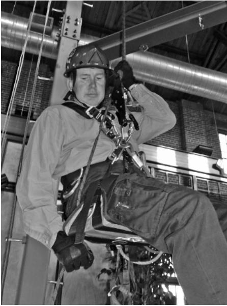
Figure 1.13 Rope access technician using a seatboard for comfort.
