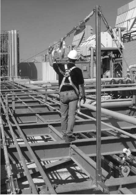
Figure 1.8 Horizontal lifeline system. Credit: Reliance Industries, LLC.
