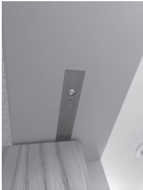
FIGURE 1.86 Center Bottom Pivot Arm (Source: Courtesy of Rixson®)
