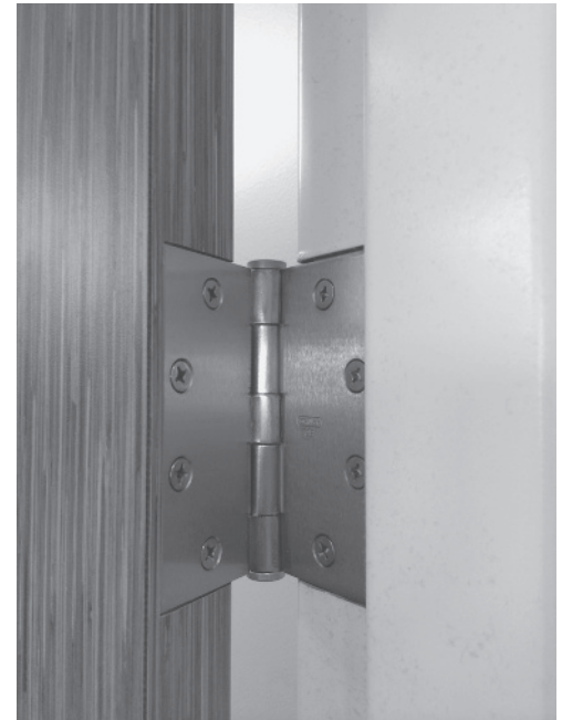
FIGURE 1.46 Full Mortise Hinge
