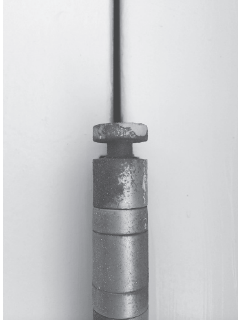
FIGURE 1.42 Rising Pin on Full Mortise Hinge Close Up (Source: Courtesy of Scott J. Tobias)
