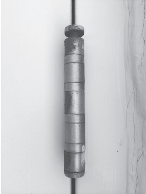
FIGURE 1.41 Rising Pin on Full Mortise Hinge (Source: Courtesy of Scott J. Tobias)
