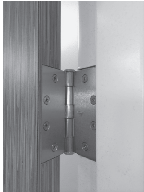
FIGURE 1.3 Nonbearing Full Mortise Butt Hinge (Source: Courtesy of Scott J. Tobias)
