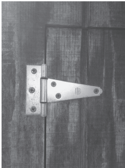
FIGURE 1.29 Tee Hinge (Source: Scott J. Tobias)
