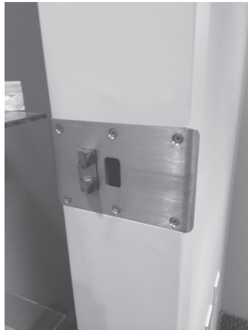
FIGURE 1.94 Double Lipped Strike with Built-In Emergency Stop
