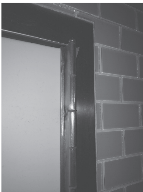
FIGURE 1.60 Pin and Barrel Continuous Hinge (Source: Courtesy of Markar Architectural Products)
