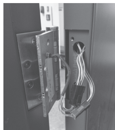
FIGURE 1.38 Molex® Connector Wired to Door (Source: Copyright © ASSA ABLOY, Inc. All rights reserved.)
