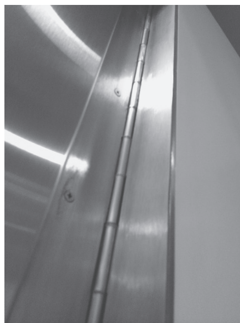
FIGURE 1.61 Pin and Barrel Continuous Hinge (Source: Courtesy of Scott J. Tobias)
