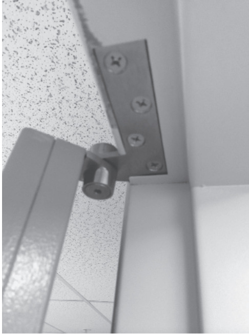
FIGURE 1.82 Offset Top-Mounted Pivot (Source: Courtesy of Rixson®)
