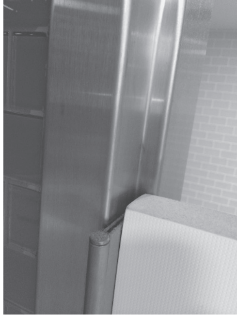
FIGURE 1.62 Pin and Barrel Continuous Hinge (Source: Courtesy of Scott J. Tobias)
