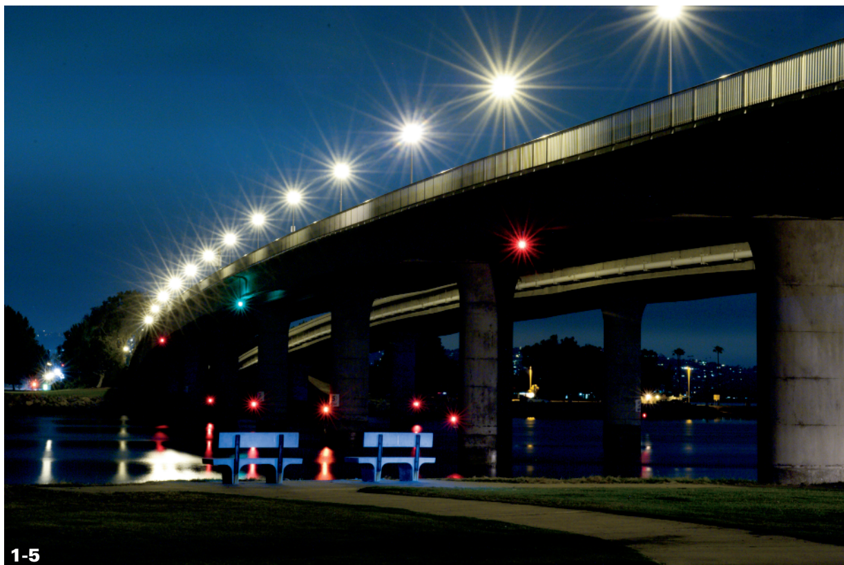
1-5 ABOUT THIS PHOTO When I took this photograph of the Ingraham Street Bridge late at night, I was limited by the light available from the bridge and needed to use a long shutter speed to capture it all. Taken at 33 seconds, f/20, and ISO 200.
