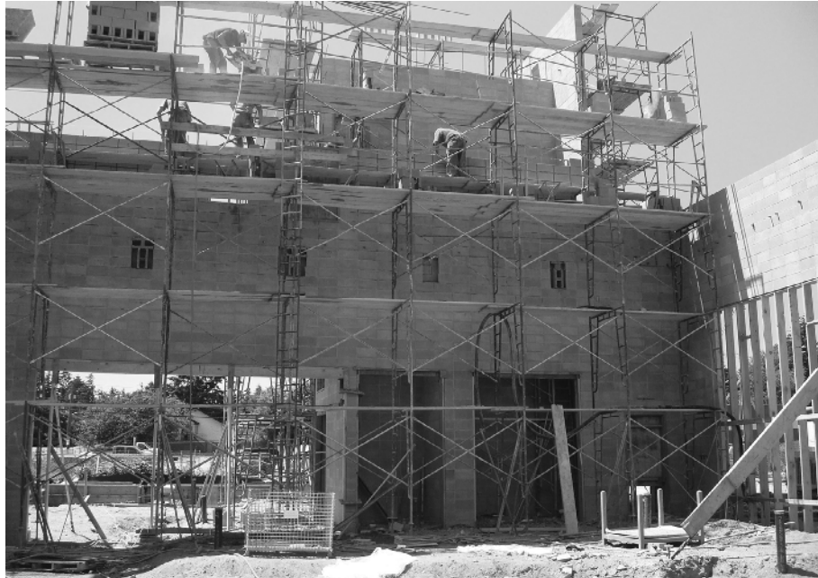
Figure 1.1 Masonry workers construct a concrete block wall from a vertical scaffold
