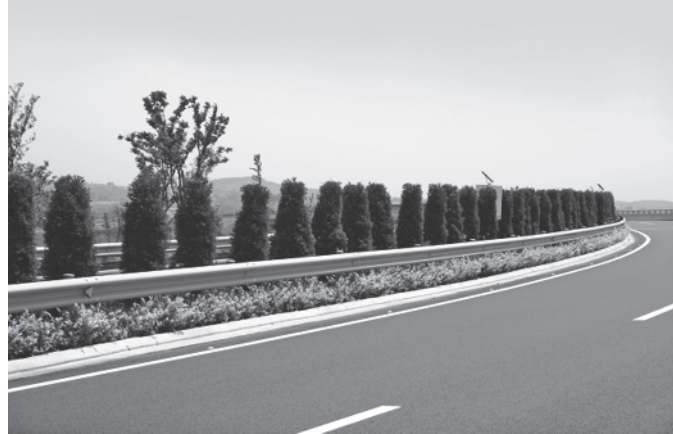
Figure 1.13 The central reservation between Luojiabian and the toll station on the main lane is 2 m wide.
