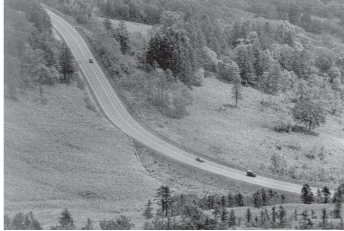
Figure 1.15 Motorway geometric design is adapted to topographical changes.
