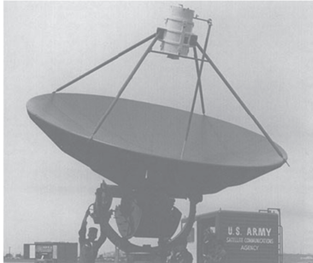
Figure 1.3 Early US Army transportable satellite communications system. Courtesy of US Army.
