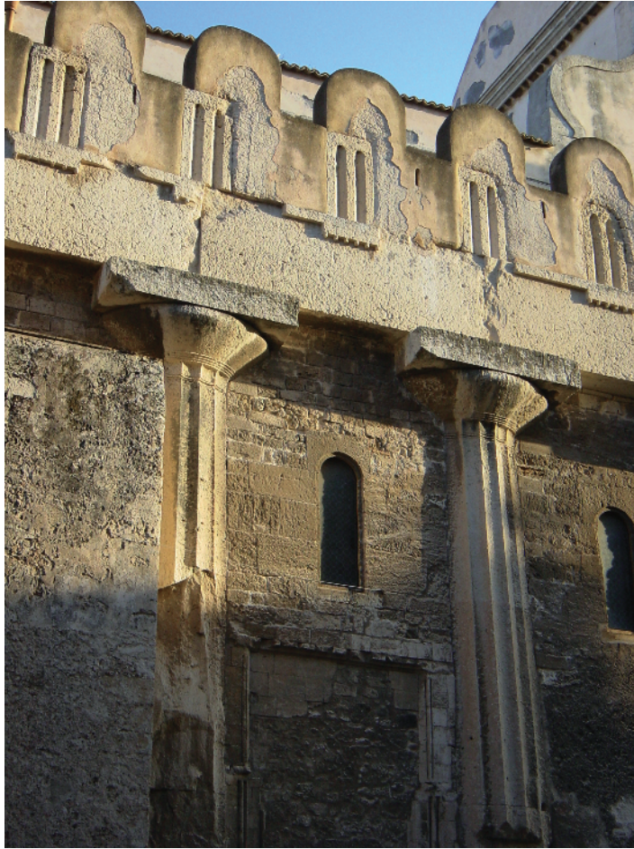
Figure 1.4 The Duomo in Syracuse, Sicily, Italy, showing elements of a classical structure incorporated into later builds of the medieval and post-medieval periods: there is no distinction between the complexity of the built fabric and its below-ground elements.
