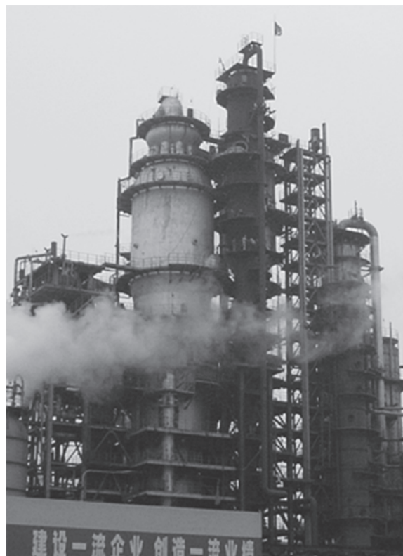
FIGURE 1.59 Profile of SRFCC in Fushun Petrochemical Company.
