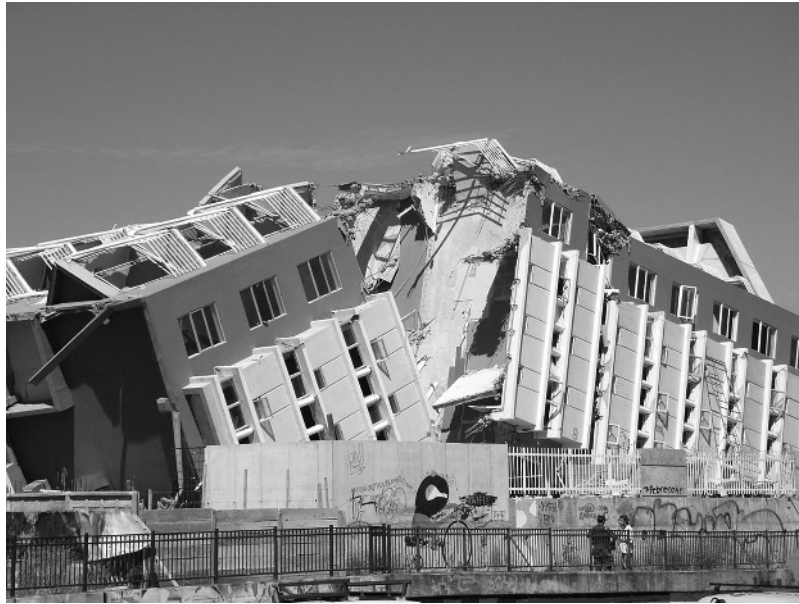
Figure 1.1 Building destroyed by a 8.8 magnitude earthquake on Saturday, February 27, 2010, with intense shaking lasting for about 3 minutes, which occurred off the coast of central Chile. (Source: Vladimir Platonow (Agência Brasil) [CC-BY-3.0-br ( http://creativecommons.org/licenses/by/3.0/br/deed.en )], via Wikimedia Commons; http://commons.wikimedia.org/wiki/File:Terremoto_no_Chile_2010.JPG )
