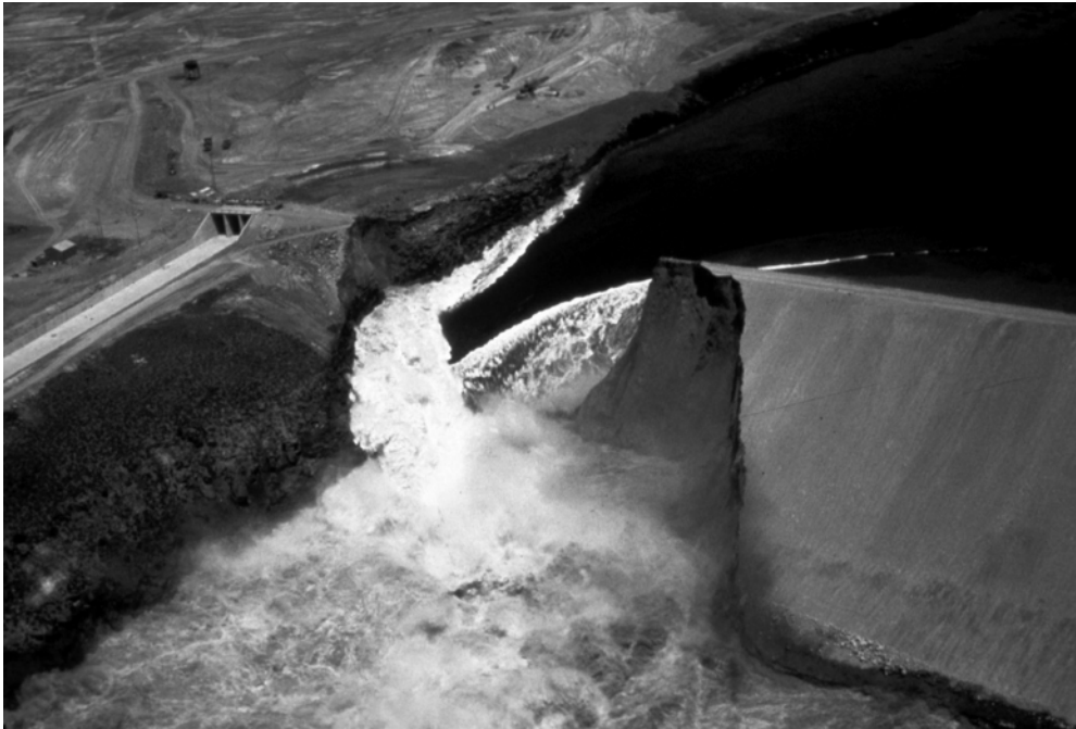
Figure 1.4 Teton Dam collapse on June 5, 1976: The collapse of an earthen dam sent a wall of water toward the Idaho Falls. The dam, located in Idaho, USA on the Teton River in the eastern part of the state, between Fremont and Madison counties, suffered a catastrophic failure as it was filling for the first time. (Source: US Government; http://commons.wikimedia.org/wiki/File:Teton_Dam_failure.jpg )
