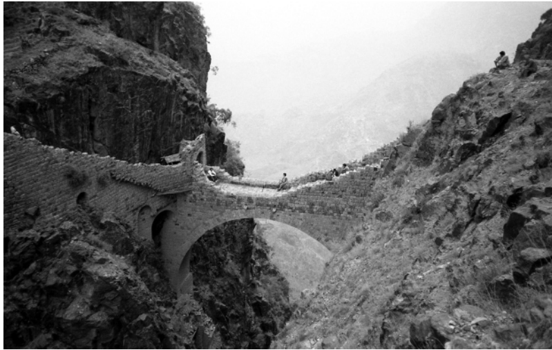
Figure 1.2 Bridge damage in Shahrarah, Yemen, August 1986. The failure of bridges is of special concern to structural engineers in trying to learn lessons vital to bridge design, construction, and maintenance. (Source: Bernard Gagnon [CC-BY-3.0-br ( http://creativecommons.org/licenses/by/3.0.en )], via Wikimedia Commons; http://en.wikipedia.org/wiki/File:Shehara_02.jpg )
