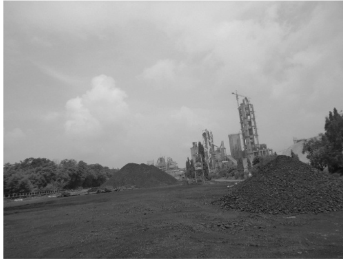
Figure 1.7 Raw material storage in cement plant.
