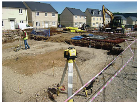
Foreman checking level of foundation concrete/ checking compact stone fill levels using the laser level
