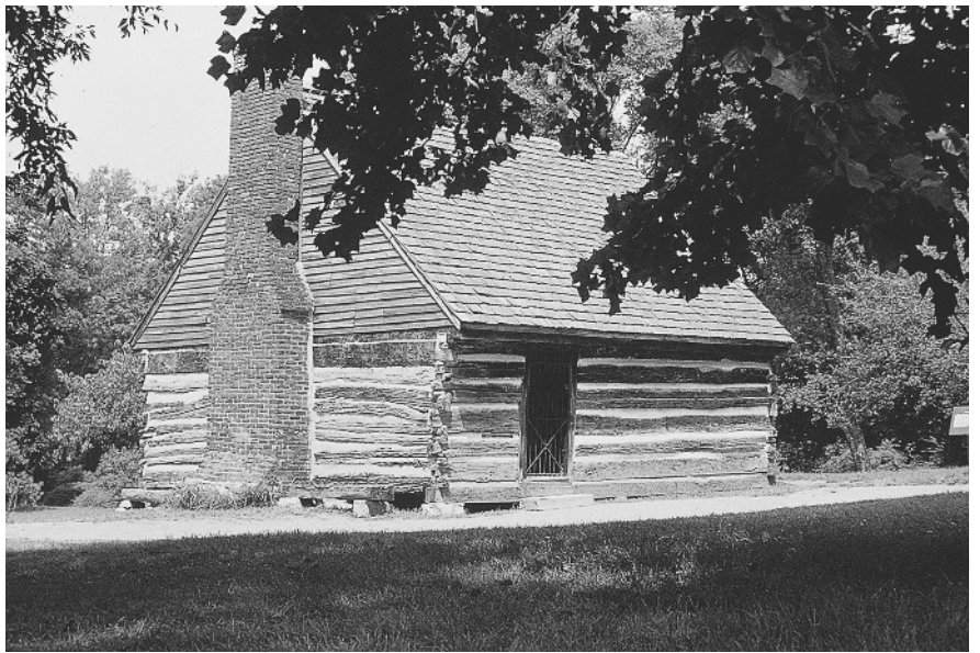
Figure 1.2f In cold climates, compactness, thick wooden walls, and a severe limit on window area were the traditional ways to stay warm. In very cold climates, the fireplace was located either on the inside of the exterior wall or in the center of the building. The log cabin was introduced to America by early Swedish settlers.
