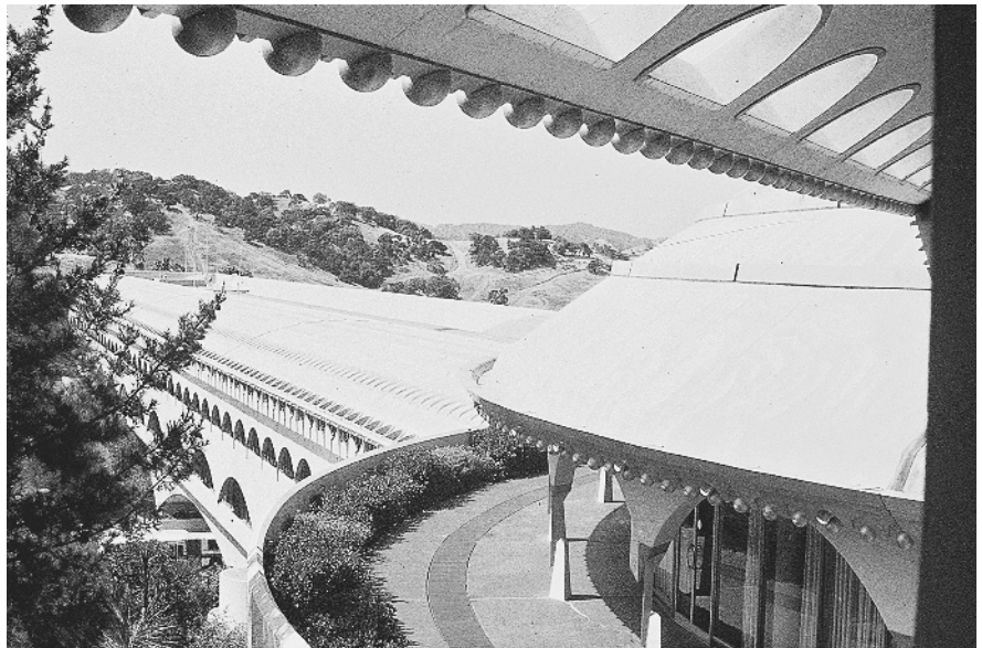
Figure 1.3f The exterior windows of the Marin County Civic Center are protected from direct sun by an arcade-like exterior corridor.
