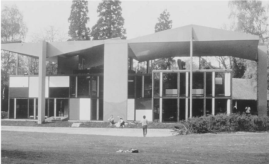
Figure 1.3g The Maison de l'Homme in Zurich, Switzerland, demonstrates the concept of the parasol roof. The building is now called Centre Le Corbusier. (Photograph by William Gwin.)
