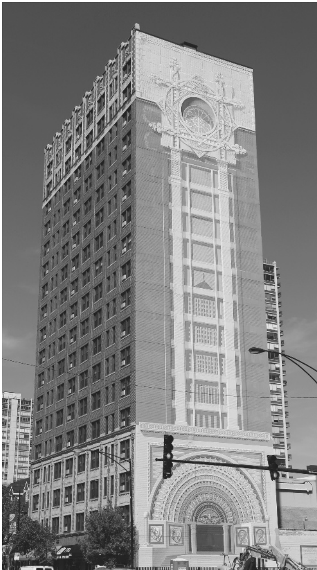
Figure 1.8 Exterior murals have become quite popular, especially in cities where the demolition of some buildings expose property line walls that were never meant to be seen. A type of mural called trompe l'oeil creates architectural illusions, as in this Chicago building. Such murals create “architecture” with a minimum of materials and energy.
