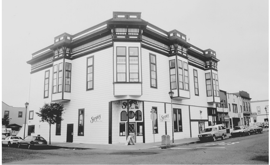
Figure 1.2e Bay windows are used to capture as much light as possible in a mild but very overcast climate such as that found in Eureka, California.
