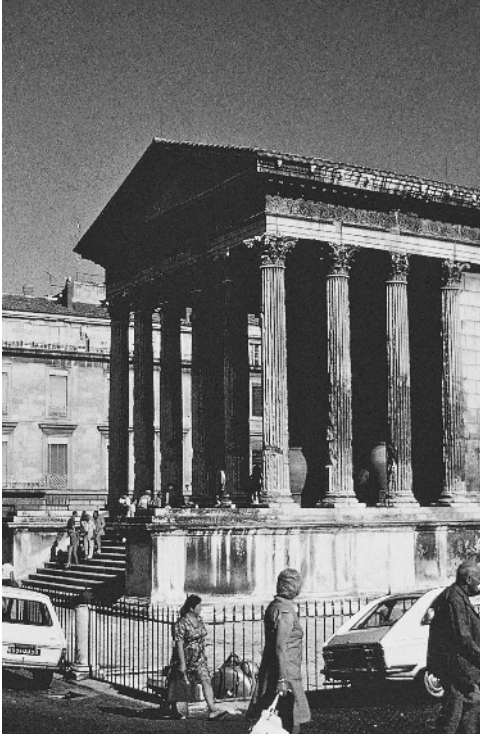
Figure 1.3a The classical portico has its functional roots in the sun- and rain-protected entrance of the early Greek megaron. Maison Carrée, Nîmes, France.
