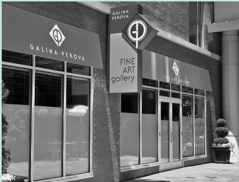
Galina Perova Fine Art Gallery, National Harbor, Maryland. Architect: K. Dixon Architecture, PLLC.
