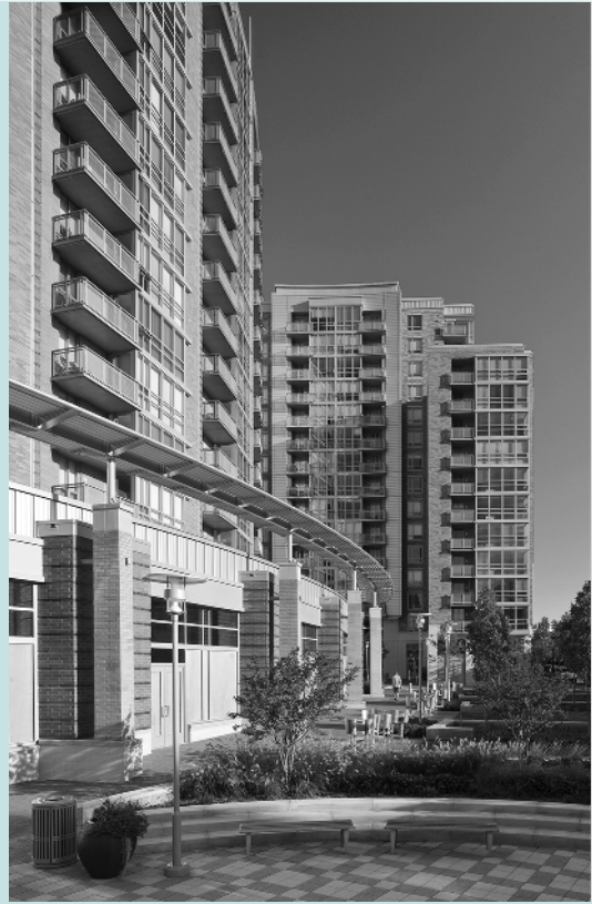
Verdian, Silver Spring, Maryland. Architect: WDG Architecture, PLLC. PHOTOGRAPHER: © MAX MCKENZIE.
