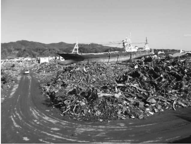
Figure 1.2 More than a dozen ships were washed inland by the Tohoku tsunami in Kesennuma City, Miyagi Prefecture. The fishing trawler Kyotoku-maru came to rest on a giant debris pile on one of the main roads to City Hall. (Courtesy of Hermann M. Fritz.)
