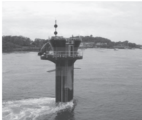
Figure 1.12 Principle of tidal energy by tidal stream generator (1.2 MW plant in Ireland) [12]
