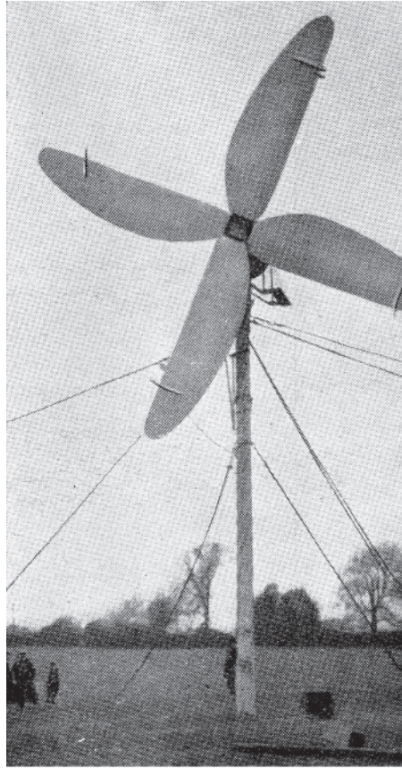
Figure 1.17 Fast-rotating wind wheel of the Aerodynamo A.G. Berlin, Kutfirstendam. The figure shows the brake flaps used by this company on the suction side of the blades [12]. Photograph originally taken by Betz, A. and used with thanks
