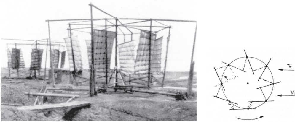
Figure 1.4 Left: Chinese wind wheels at Taku that pump brine solutions for the extraction of salt (Hopei [3]). Reproduced with permission of E & F N Spons; right: schematic depiction of the function of a Chinese windmill. Solid lines represent blades and dash-dotted lines represent sails [5].
