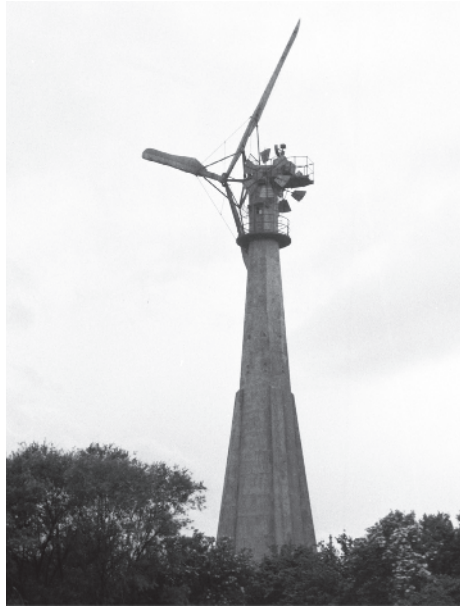
Figure 1.20 An out-of-service Smidth-Aeromotor in Denmark. Rotor diameter 24 m, nominal output approximately 70 kW. Photo by Paul Smulders in 1972
