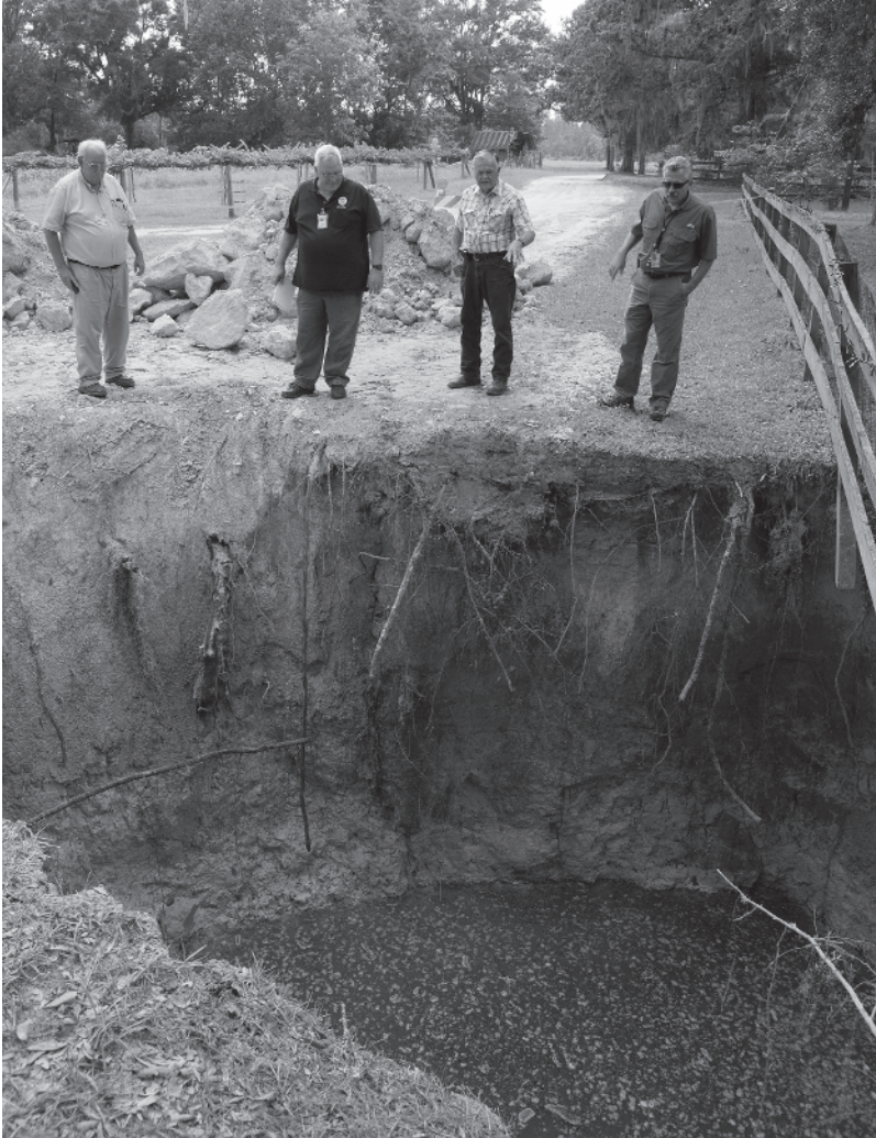
This 45 foot-deep sinkhole formed in Monticello, FL, after Tropical Storm Debby produced excessive rains and flooding. David Fine/FEMA.
