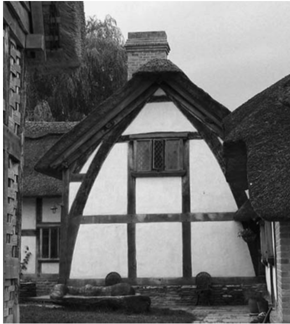
Figure 1.1: Photograph of typical cruck construction in Herefordshire.
