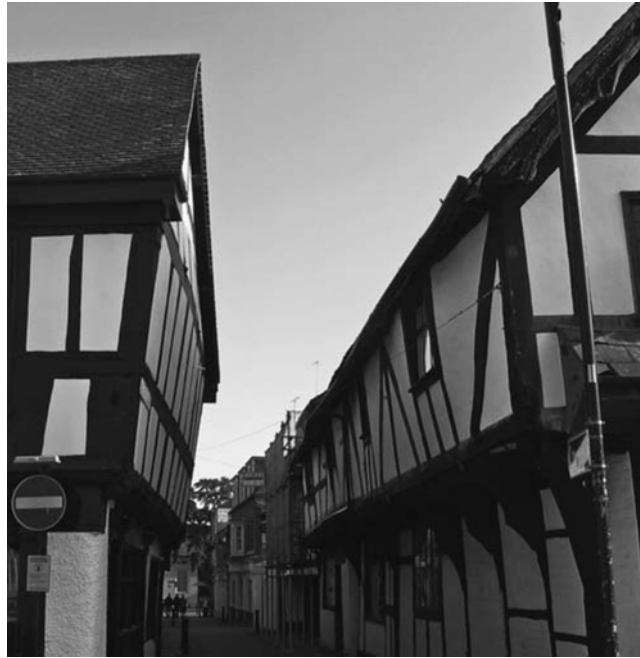
Figure 1.2: Photograph showing the close proximity of timber frame housing in Leominster, increasing the risk of fire.
