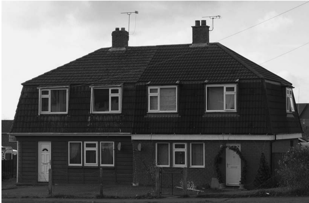
Figure 1.10: Photograph of a Cornish dwelling which was a particular type of prefabricated concrete house.
