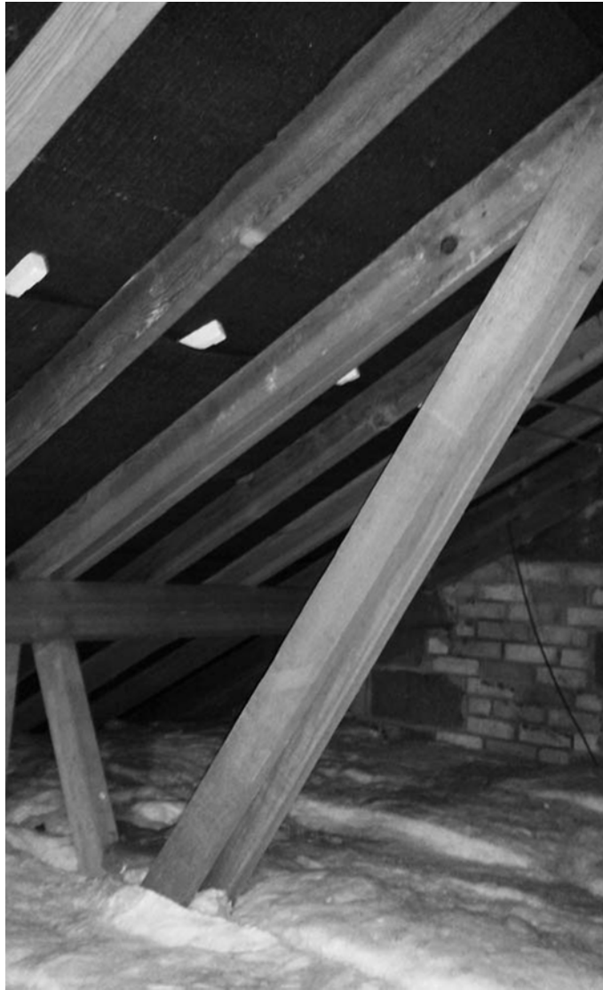
Figure 1.11: Photograph of a TRADA truss.
