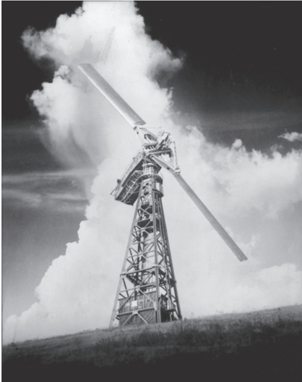
FIGURE 1.22 The 1.25 MW Smith–Putnam Wind Turbine of 1942, the first utility-scale, grid-connected wind turbine in the United States ( Photo from the archive of Carl Wilcox in the possession of Paul Gipe).
