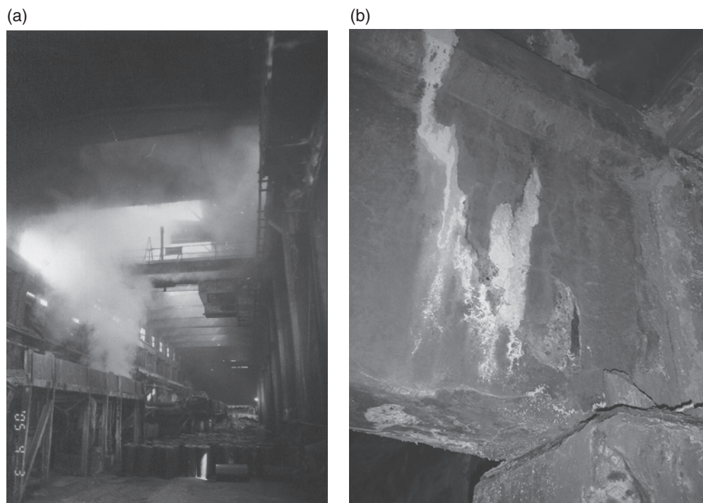
Figure 1.2 Advanced deterioration of concrete elements in a steel process workshop constructed in 1980, aged 24 years at inspection. The RC elements in the steel workshop were exposed to high concentration of corrosive gas rich in chloride and sulfate, high temperature, and humidity (a). The local degradation was manifested through advanced corrosion of steel bars, concrete spalling, and leachates from concrete cracks (b). Source: courtesy of Tingyu Hao.
