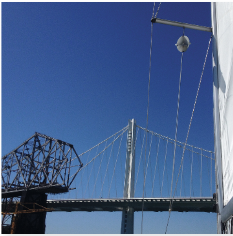
Charles Henry Purcell, San Francisco-Oakland Bay Bridge, Oakland, California, 1937
