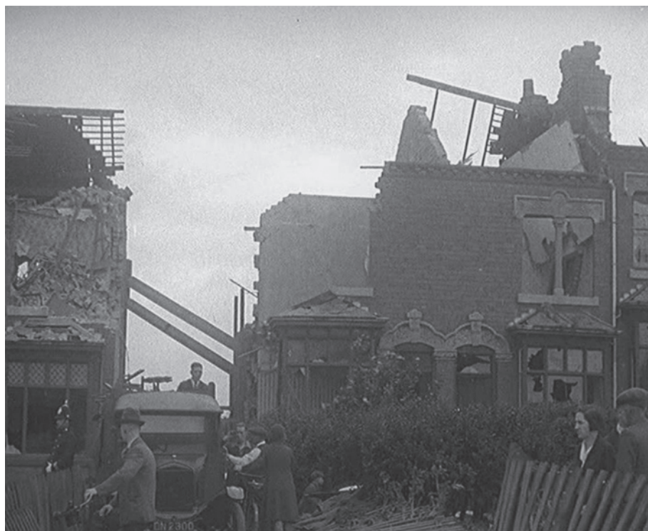
Figure 1.11 Structural property damage as a result of the Birmingham tornado of 14 June 1931. Shops and houses on the Coventry Road received severe damage. © British Pathé.
