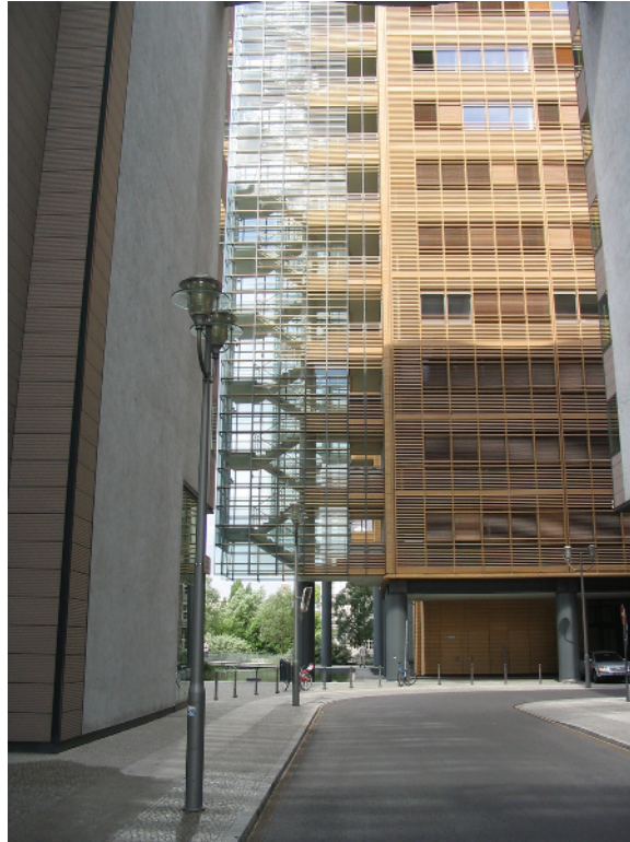
Fig. 1.3 A very visible staircase. How is it supported? You'll learn more about cantilevers later in the book.
