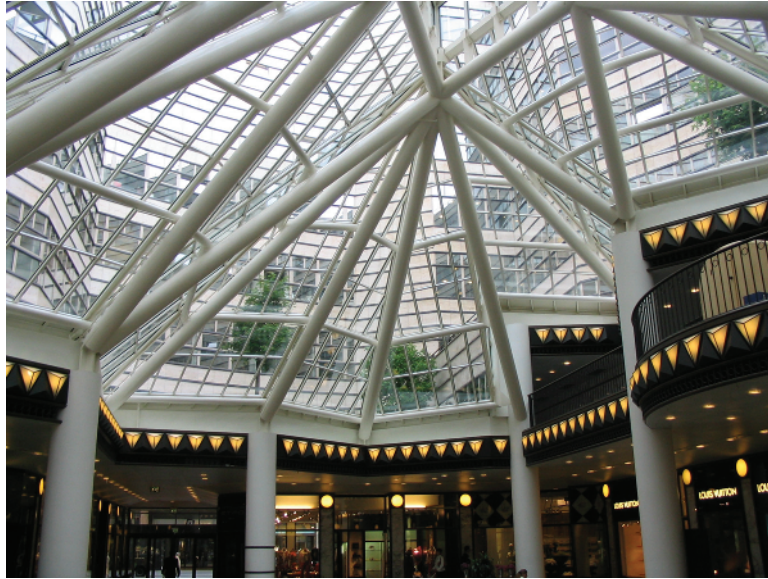
Fig. 1.2 Roof structure of Quartier 206 shopping mall, Berlin. Quite a 'muscular' roof structure!
