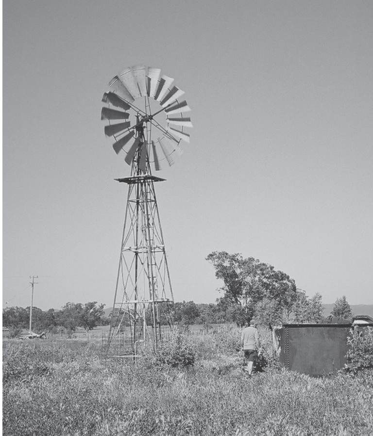
Figure 1.4 Drilled well fitted with a windmill pump used for livestock watering, New South Wales, Australia. Photo by Bruce Misstear
