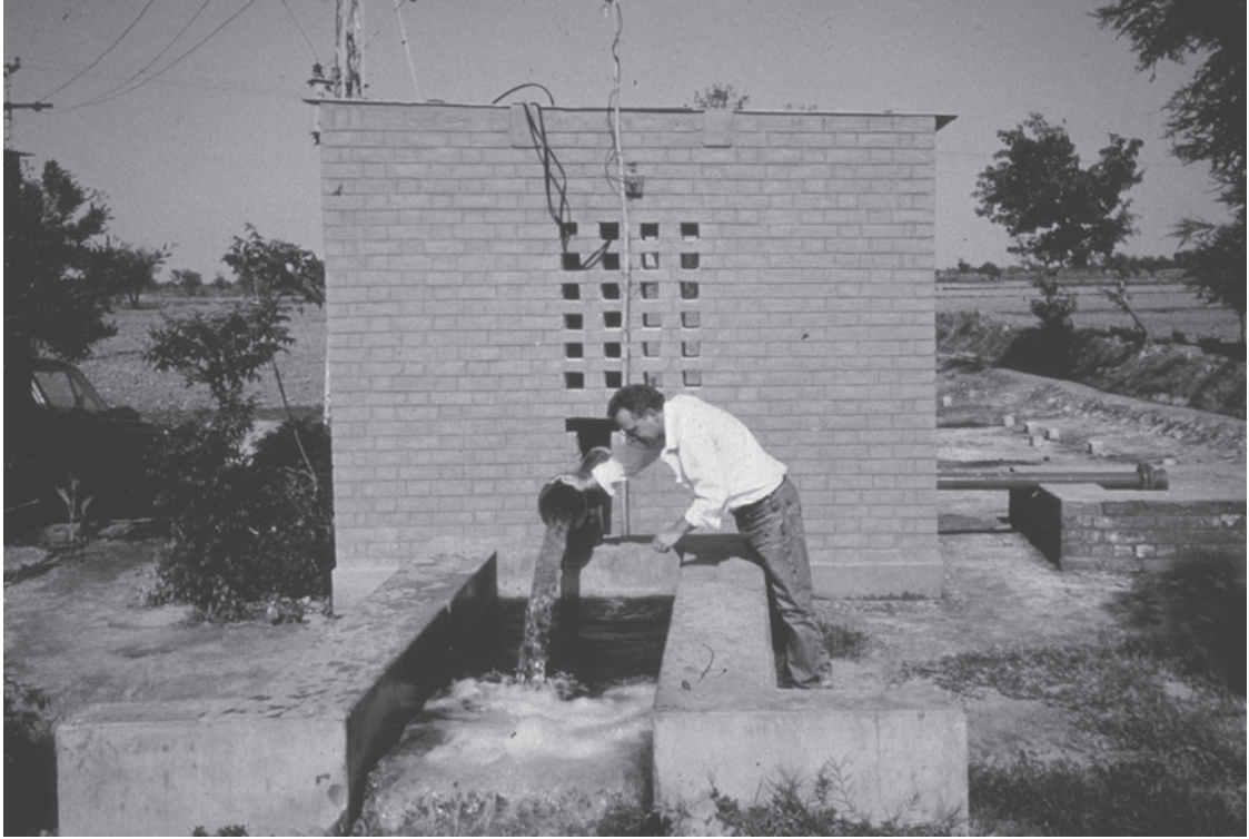
Figure 1.3 A dual purpose irrigation and drainage well in the Indus valley, Pakistan. In this ‘scavenger well’ the outlet pipe in the foreground of the picture is discharging fresh groundwater from the upper part of the well, whereas the pipe to the right is discharging saline water from the lower section of the well, thus preventing the saline water from moving upwards and contaminating the good quality water. The good quality water is used for irrigation whilst the saline water is diverted to the drainage system. Photo by Bruce Misstear
