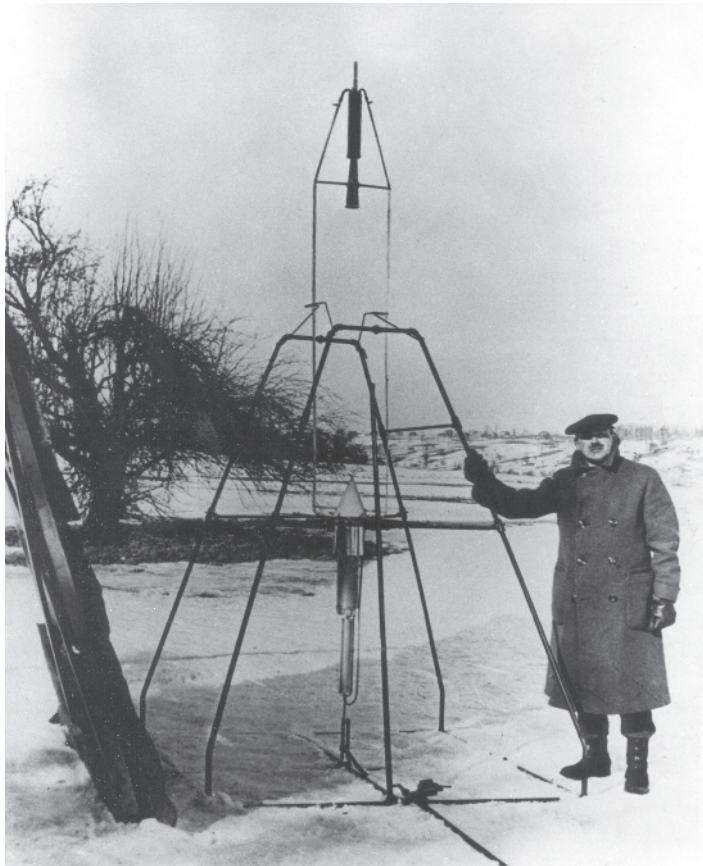
Figure 1.75 Robert Goddard with the first liquid-propellant rocket (Goddard is holding the trapezoidal launch frame). (Source: NASA.)
