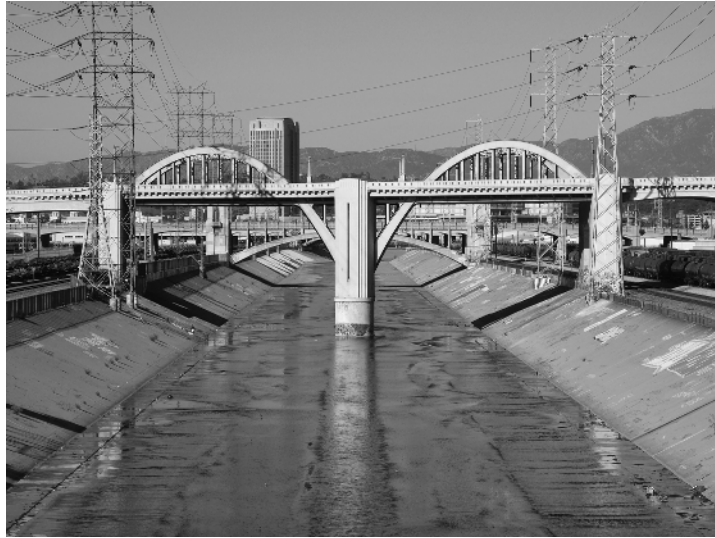
FIGURE 1.1 The highly engineered drainage system of the Los Angeles River exemplifies the almost total degradation of a natural riparian system.
