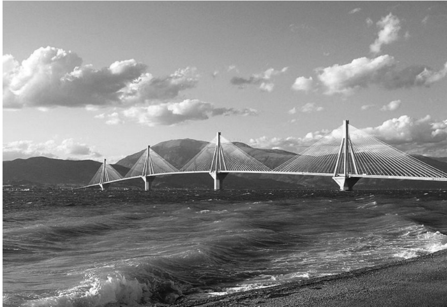
FIGURE 1.3 The Charilaos Trikoupis bridge in Greece, with a sensor network installed with over 300 sensor nodes. In its first days, it signaled abnormal vibrations, which could be quickly fixed. Source: Guillaume Piolle, Flickr.
