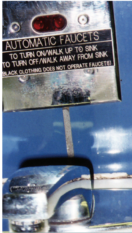
Figure 1.10 A sign in the restrooms at Cincinnati airport. Because it is not visible to the user as to what to do to turn the faucet (tap) on and off, a sign has been added to explain what is normally an everyday and well-learned activity. It does not explain, however, what to do if you are wearing black clothing
