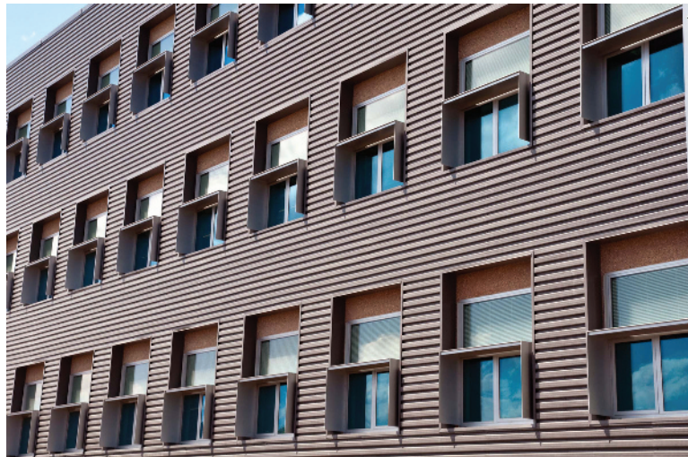
Figure 1.7 (D) The fenestration for the NREL RSF was designed to provide excellent daylighting while controlling glare and unwanted solar thermal gain through the use of shading devices, recessed windows, and electrochromic glass. Operable windows allow the occupants to control their thermal comfort and obtain fresh air. (Source: National Renewable Energy Laboratory)
