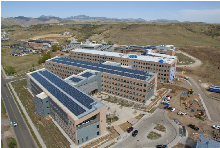
Figure 1.7 (A) The NREL Research Support Facility in Golden, Colorado, is a four-story NZE building that combines low-energy design with high-efficiency photovoltaics to produce all the energy it requires over the course of a year. (Source: National Renewable Energy Laboratory)
