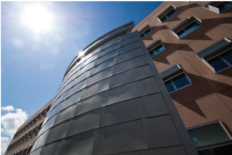
Figure 1.7 (B) Ground view of the air intake structure that conducts outside air into the thermal storage labyrinth in the crawl space of the NREL RSF. (Source: National Renewable Energy Laboratory)
