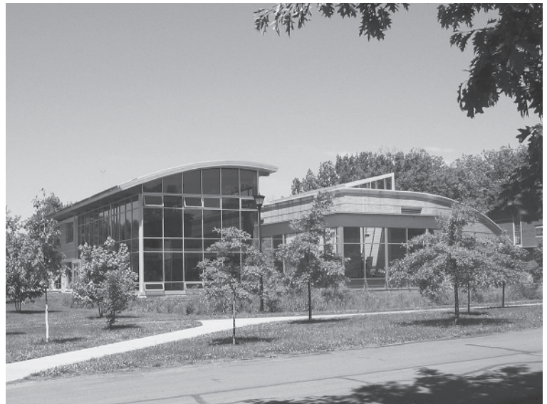
Figure 1.6 The Lewis Center for Environmental Studies at Oberlin College in Oberlin, Ohio, was designed by a team led by William McDonough, a leading green building architect, and including John Todd, developer of the Living Machine. In addition to the superb design of the building's hydrologic strategy, the extensive PV system makes it an NZE building. (Photograph courtesy of Oberlin College)
