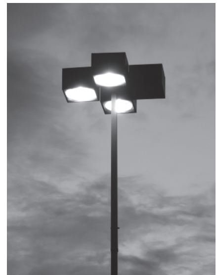
Figure 1.3 Understanding what we see leads to better energy improvements.
