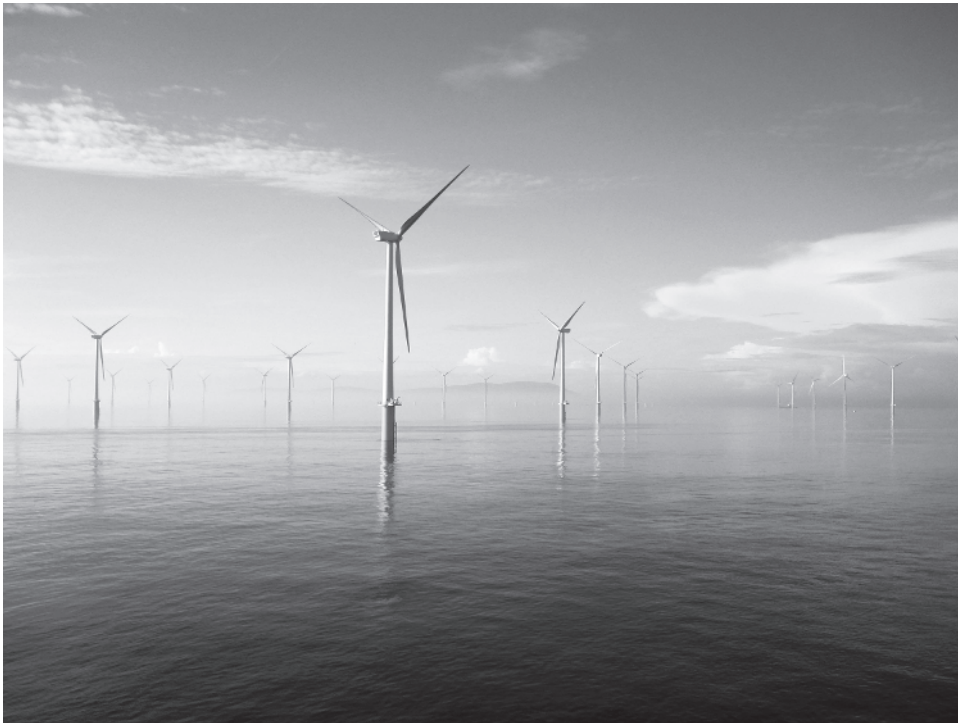
Figure 1.3 The London Array 630-MW offshore wind farm in operation in the outer Thames estuary. The wind farm spans about 100 km 2 and includes 175 turbines each rated 3.6 MW installed in waters up to 25 m deep (London Array Limited, 2016). Source: London Array Limited.
