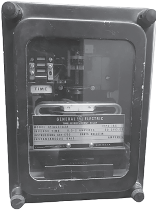
Figure 1.26 Electromechanical relay for overcurrent protection.
