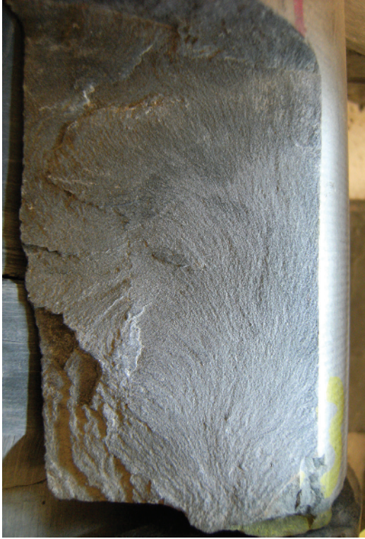
Figure A1b1.8 A wandering plume structure on the face of an extension fracture propagated upward, oblique to the core axis in a limestone. Plume axes parallel to the core axis suggest coring-induced fractures, but this fracture is natural as suggested by the upward vs downward growth of the plume and its asymmetry relative to the core axis. The fracture terminates at the top at a shalier unit. Vertical four-inch diameter core, uphole is towards the top of the photo.
