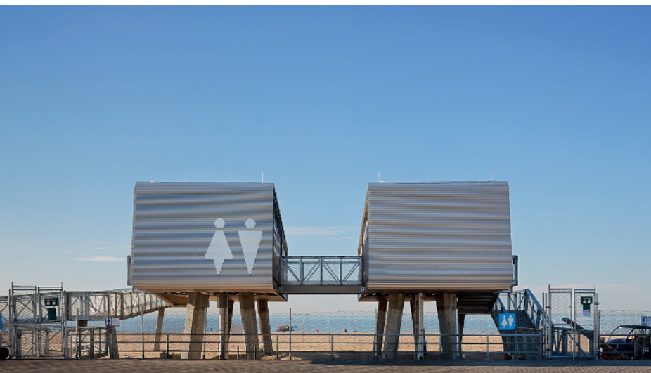
1 Garrison Architects, New York City Beach Restoration Modules, New York, USA, 2013. The section shows building elements and systems. The modules are raised on concrete legs to withstand significant sea level rise.
