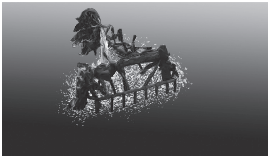
Figure 1.16 Burnt out of Bombay High North platform
