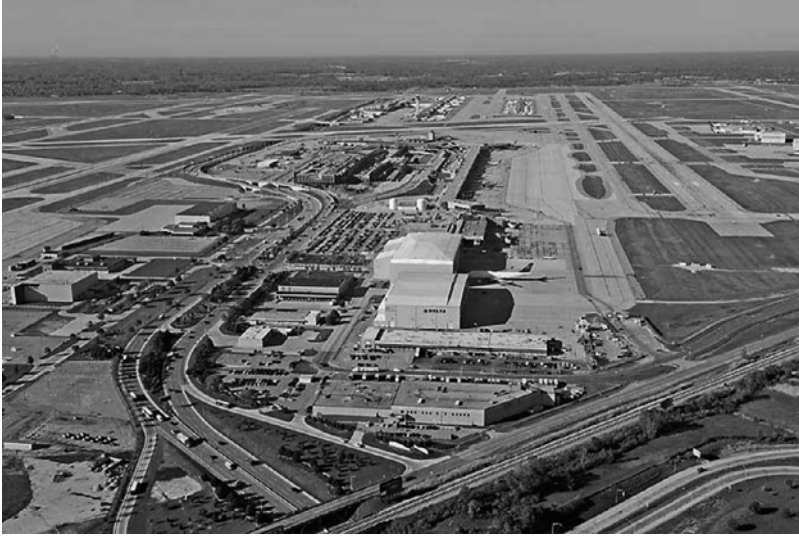
Figure 1.1 An aerial view of Hartsfield–Jackson Atlanta International Airport.
