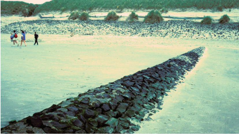
Figure 1.9 Large groyne to protect the beach from erosion on the North Sea coast of the Netherlands. There is a small dike landward of the dry beach.
