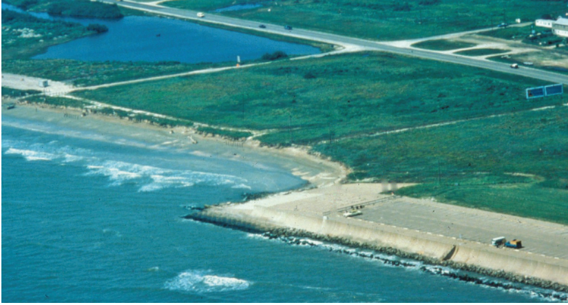
Figure 1.10 South end of the Galveston sea wall on the Texas coast showing how it is protecting the shoreline from erosion.
