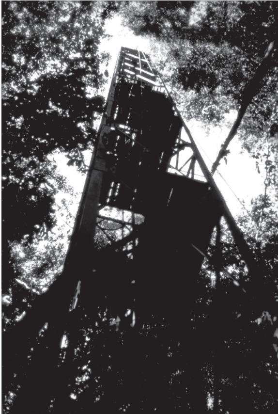
Figure 1.2 Details of the steel tower used as a platform to collect mosquitos, and to keep the caged monkeys in the Zika Forest. The platforms can reach the canopy of the trees. Obtained from the University of Glasgow (AJ Haddow and University of Glasgow Archives & Special Collections, Papers of AJ Haddow, GB248 DC 068/80/62).
