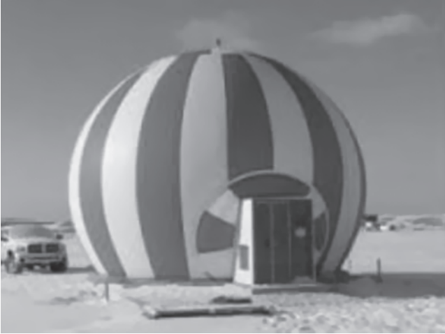
Figure 1.5 A typical inflatable radome.
