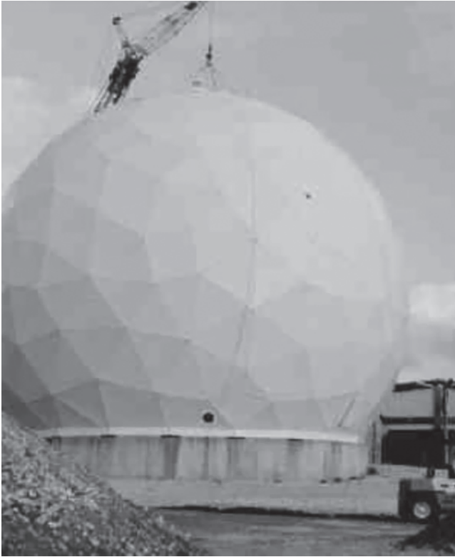
Figure 1.8 Dielectric space frame radome of AFC, Ocala, Florida.
