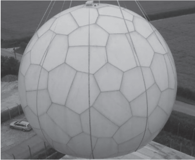
Figure 1.6 Multipanel sandwich radome of L-3 Communications-ESSCO, Concord, Massachusetts.
