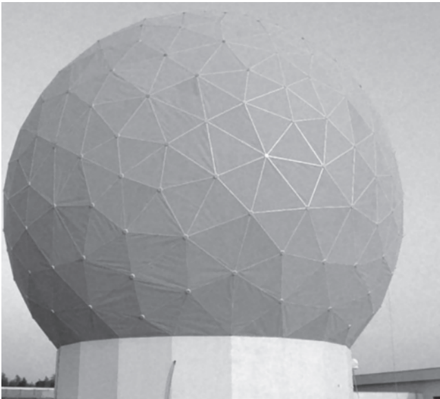
Figure 1.7 Metal space frame radome of L-3 Communications-ESSCO, Concord, Massachusetts.
