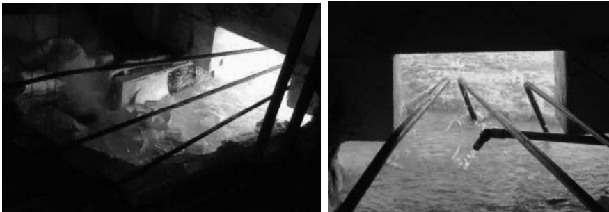
Figure 20. Water Lances Placed via. the GLB Opening
