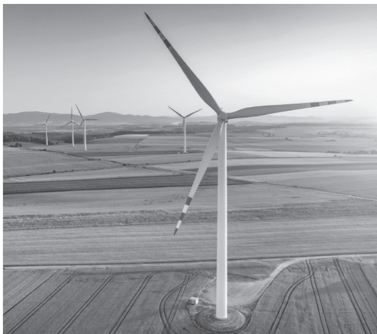
Figure 1.4 Onshore wind turbines in flat terrain. Source: Stockr/Shutterstock.com.
